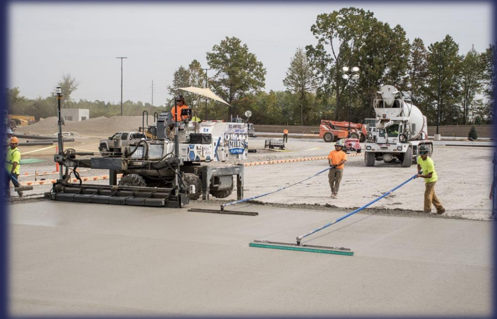
Photo Shows a 3-D Laser Screed in Action
