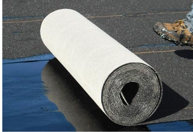
Modified Bitumen Roofing
