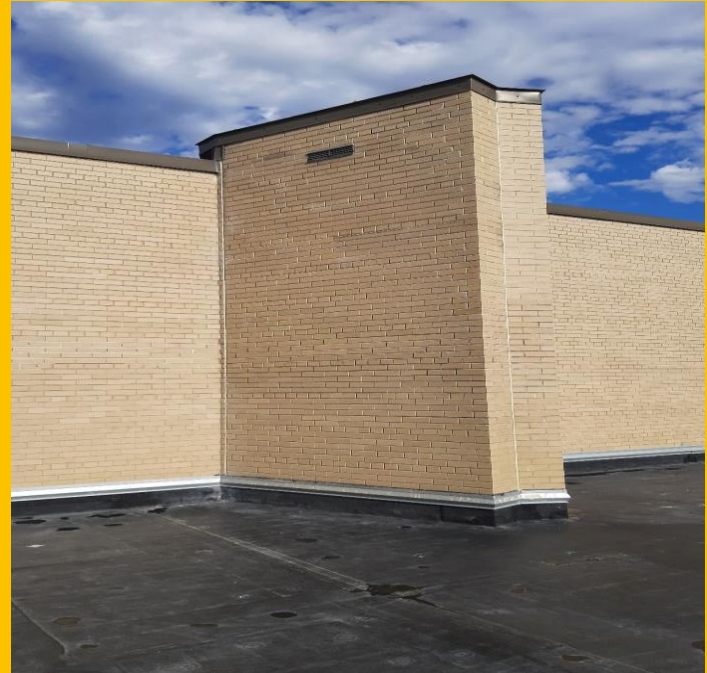
Completed Brick Replacement
