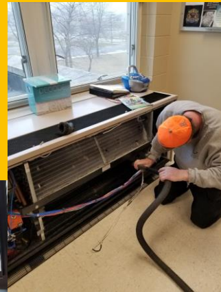
Uni-Vent Cleaning/ Bearing Repair
