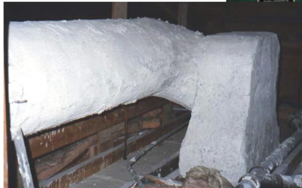
TROWELED-ON INSULATION ON KITCHEN HOOD EXHAUST DUCT
