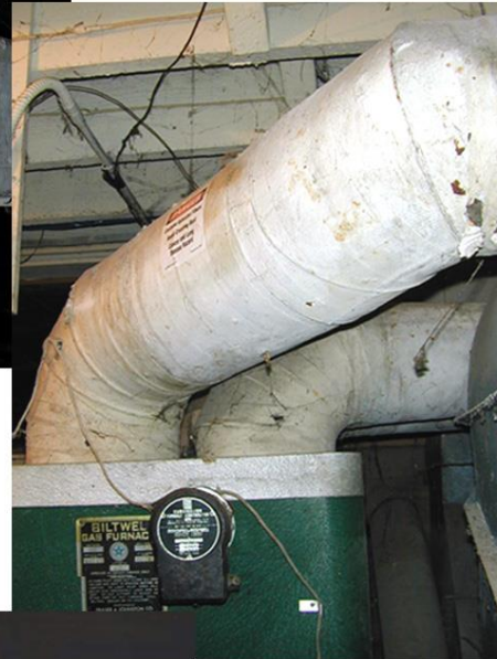
CORRUGATED (ABOVE) AND FLAT (RIGHT) ASBESTOS PAPER ON FURNACE DUCTS
