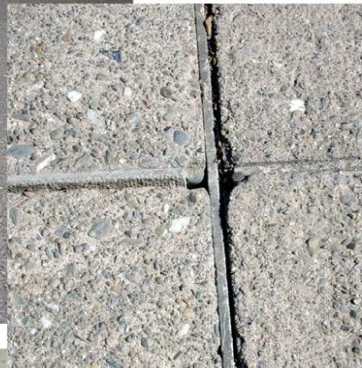
BENDERBOARD BETWEEN CONCRETE PAVERS (TRESIDDER STUDENT UNION)
