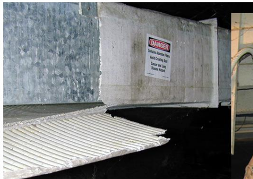
CORRUGATED (ABOVE) AND FLAT (RIGHT) ASBESTOS PAPER ON FURNACE DUCTS
