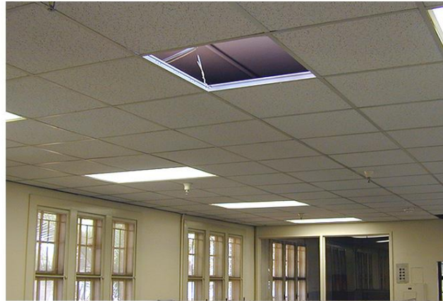
LAY-IN ACOUSTIC CEILING TILE
