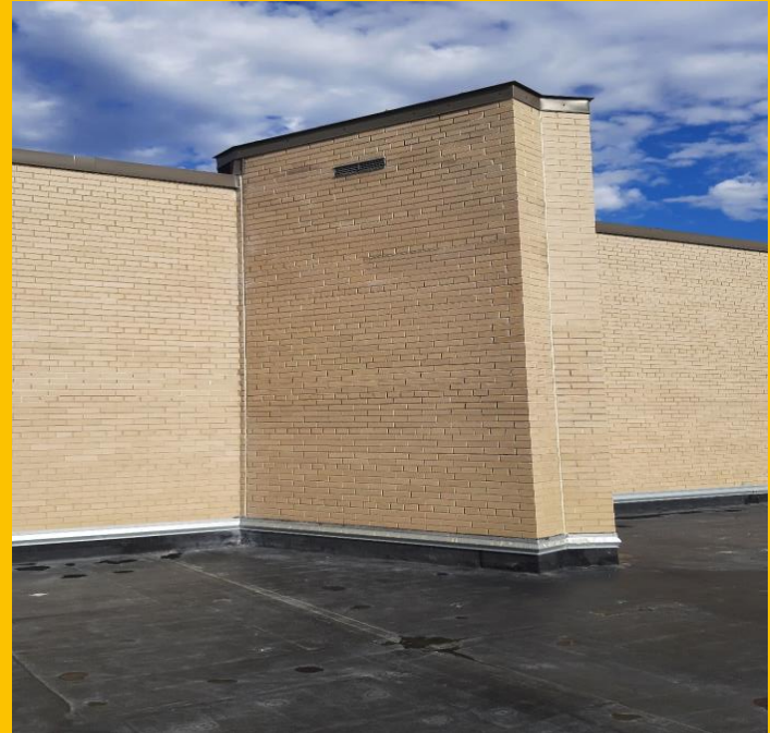
Completed Brick Replacement
